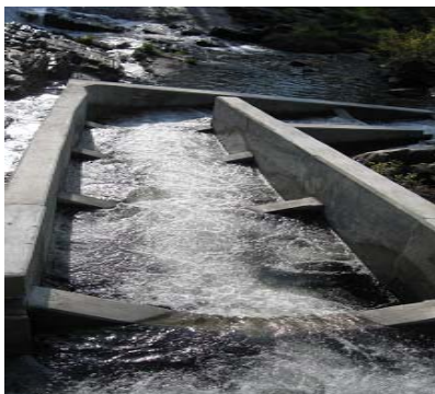
Figure 1 - Granlees North Fish Ladder
