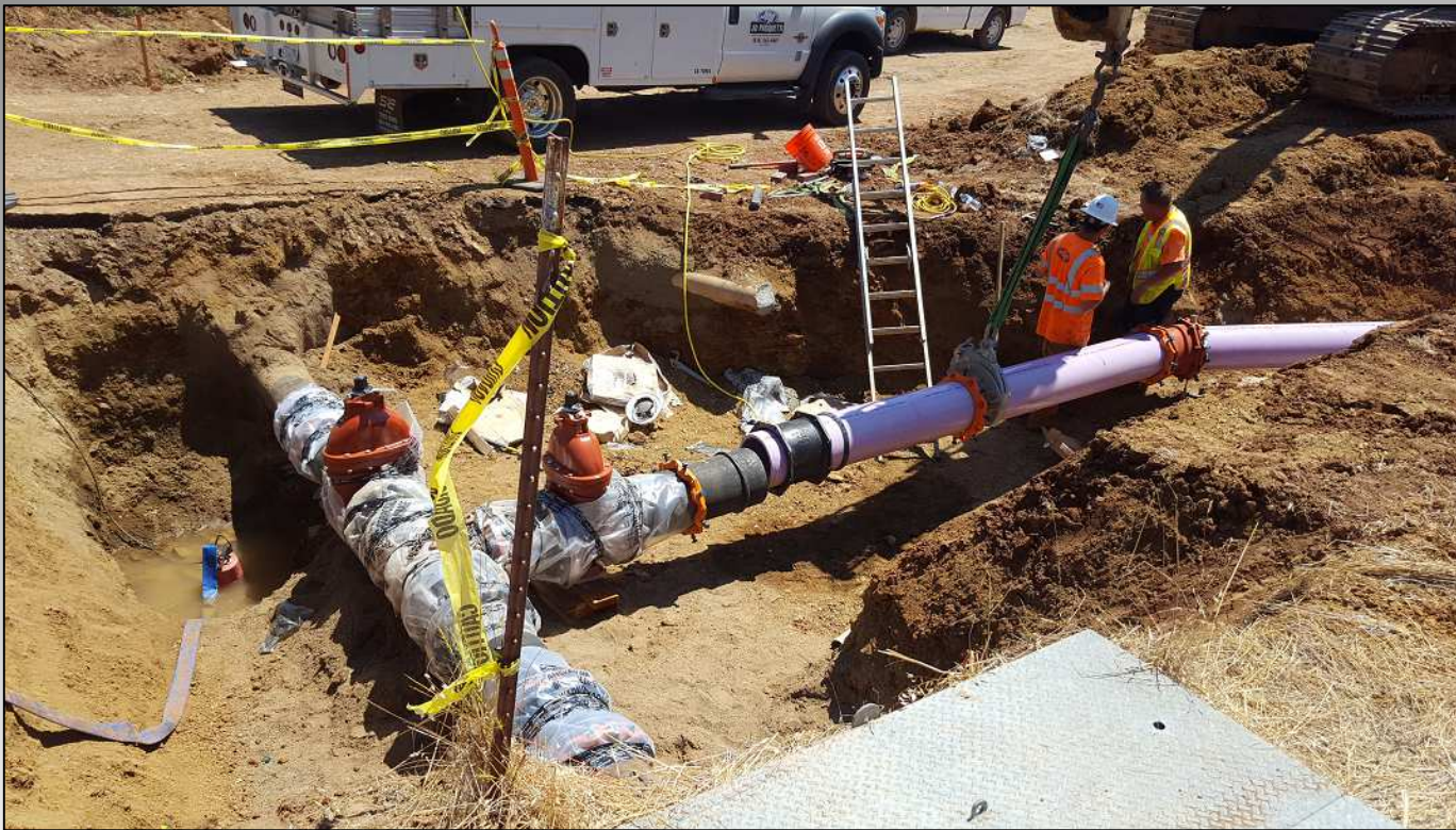
Photo of point of connection from recycled water line going to Bass lake to Murieta Gardens/Commercial areas Boring under Highway 16
