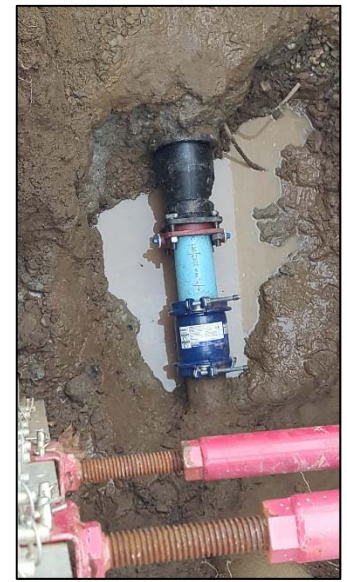
Final repair made by District
