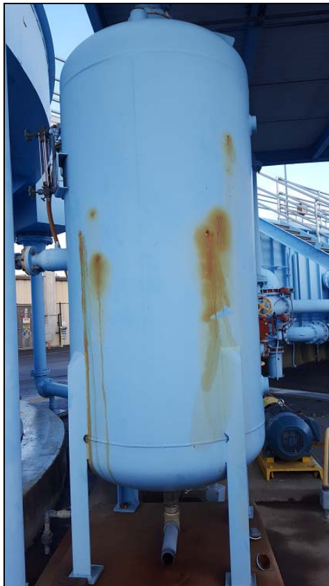
Photo of West DAF saturation tank
