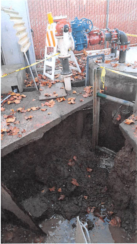
Photo 1: Trench excavation at force main break, illustrating sloughing of trench under existing AC , dated 12/17/18.
