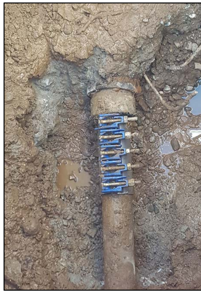
Temporary repair made with District's stainless-steel repair band
