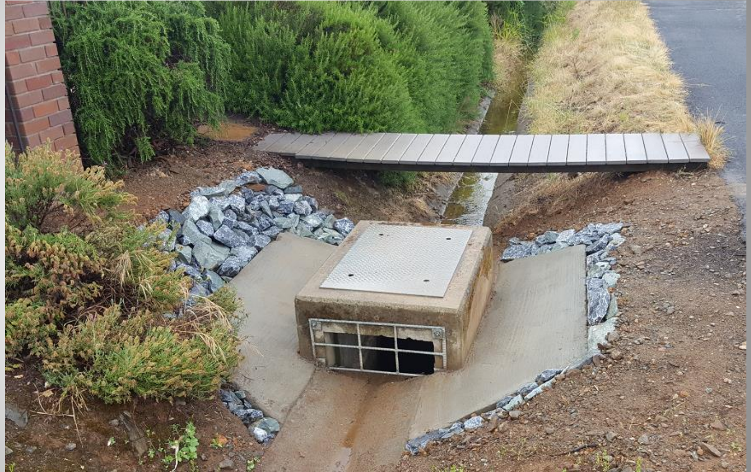
Chesbro drain repair.
