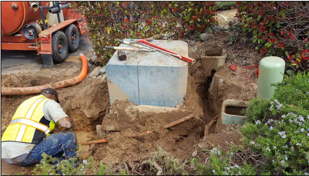
Utility Staff replacing a water service line around SMUD transformer
