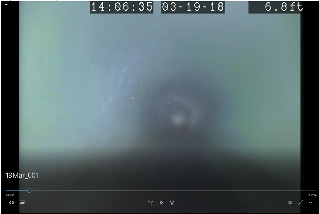
Capture #10: Beyond area of failure toward sewer main (further)
