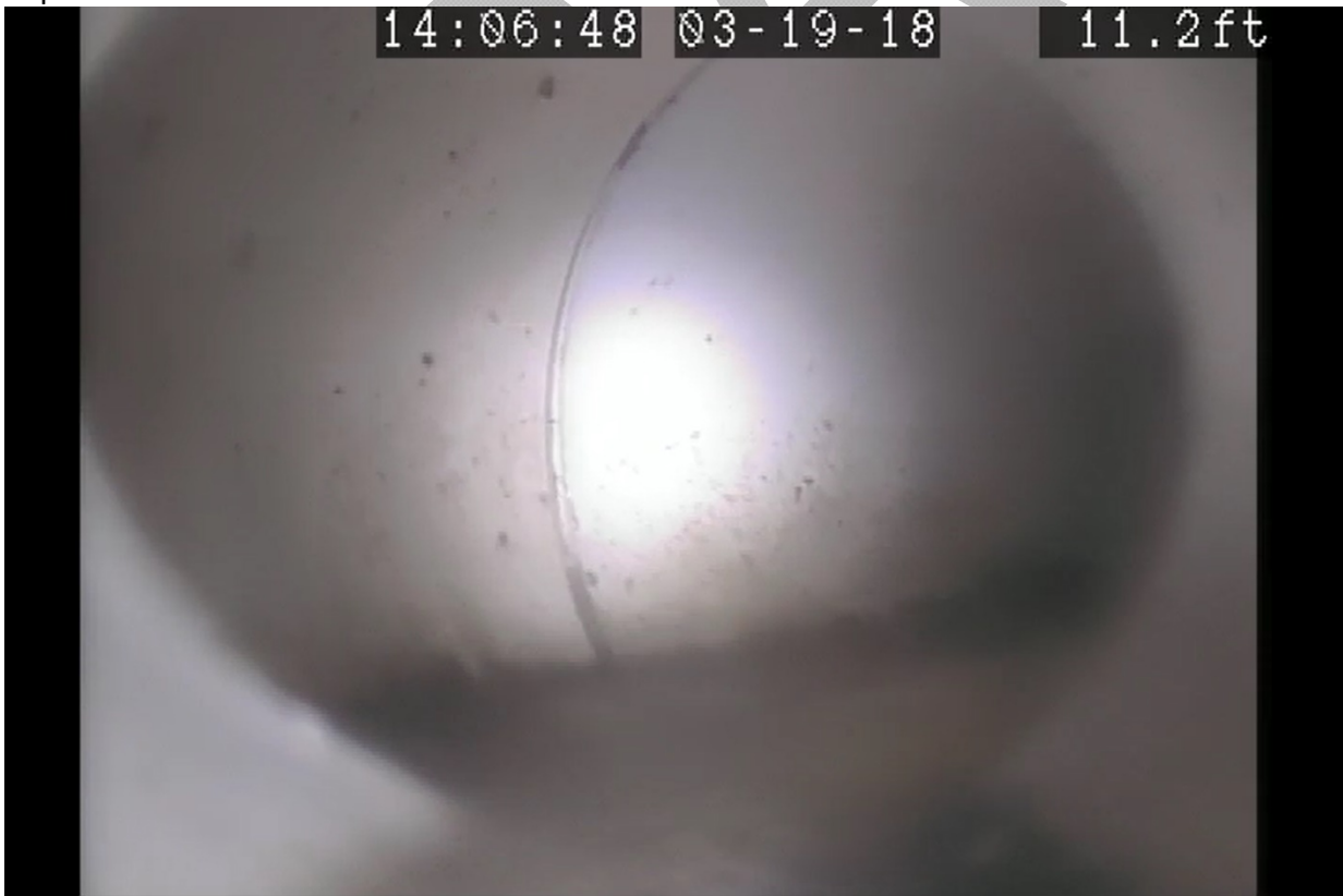
Capture #15: Clear shot of sewer main
