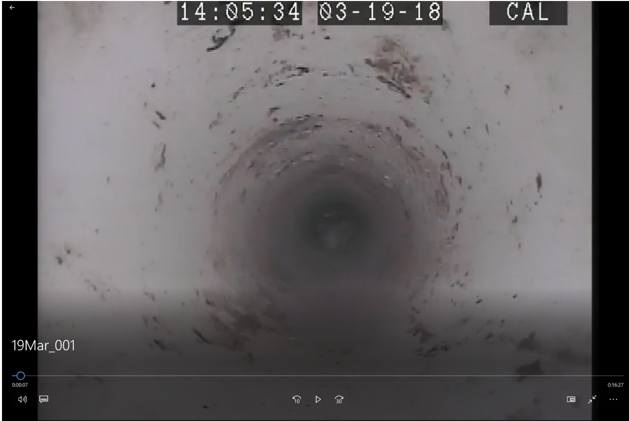
Capture #1: Scope being lowered down shaft of cleanout (note absence of effluent along pipe)
