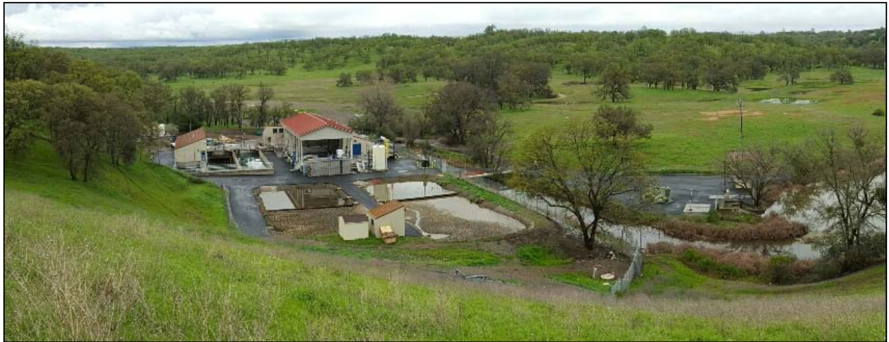
Overview of Water Treatment Plants from Chesbro Dam showing paving around facility
