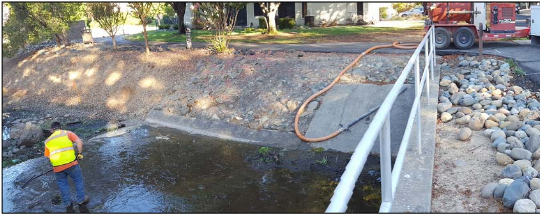
Photo of Utility staff cleaning up inlet to Laguna Joaquin
