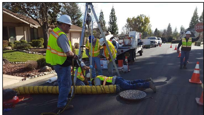
Staff working with contractor to stop I&I in a manhole
