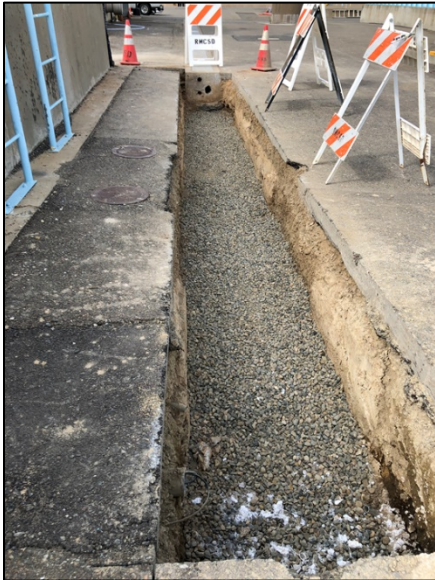
Chemical trench and trench boxes being readied for installation
