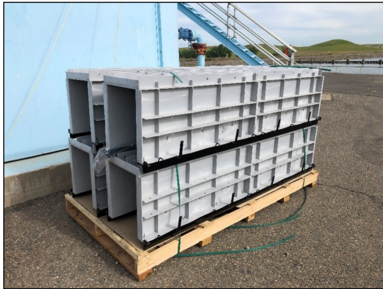
Chemical trench and trench boxes being readied for installation
