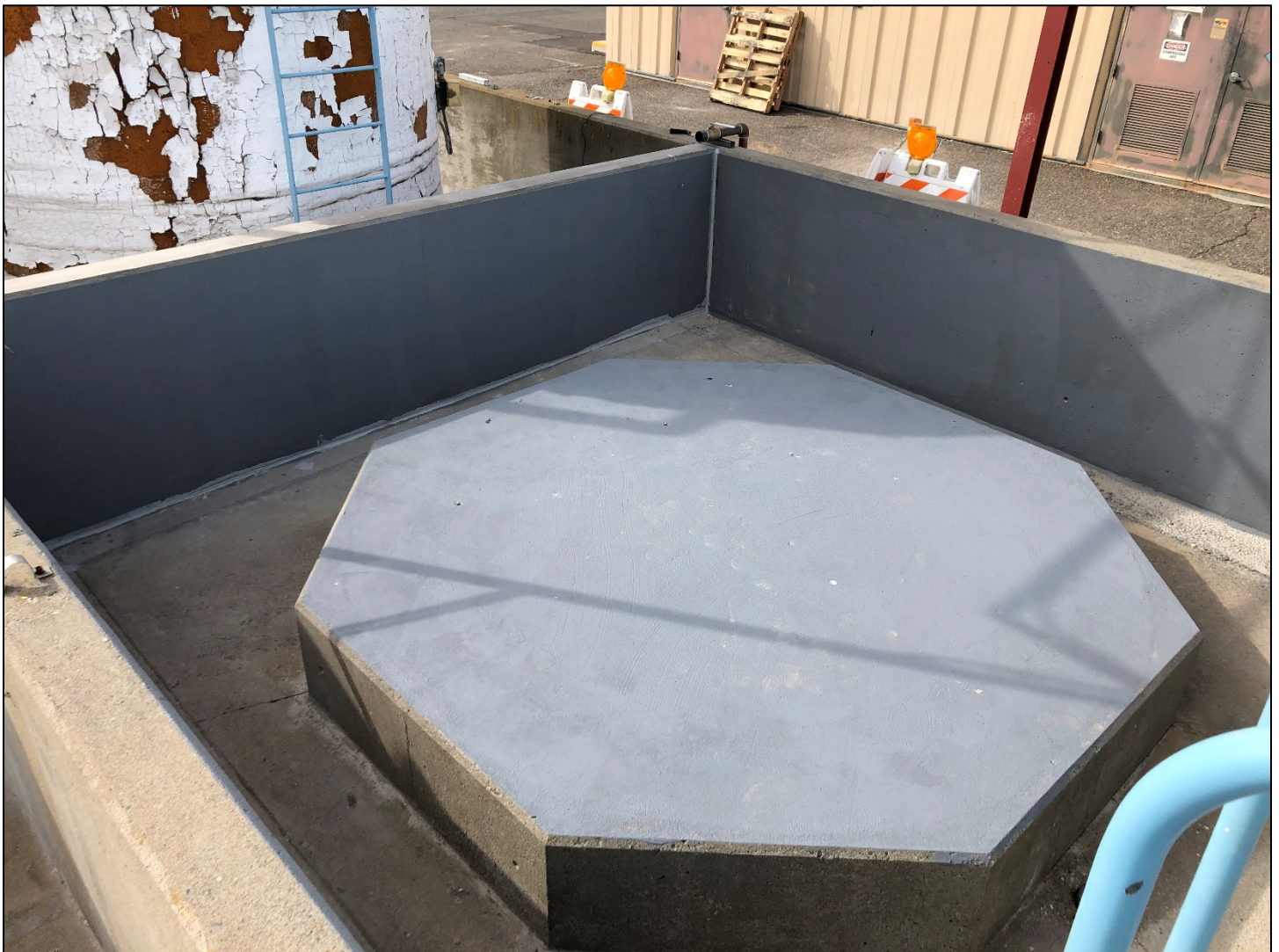
Beginning work of Epoxy painting of chemical tank area
