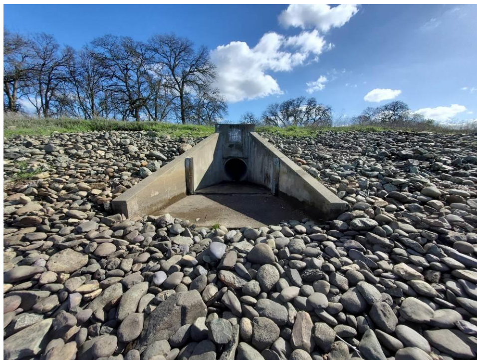
Photo 7: View of the spillway approach and control section.
