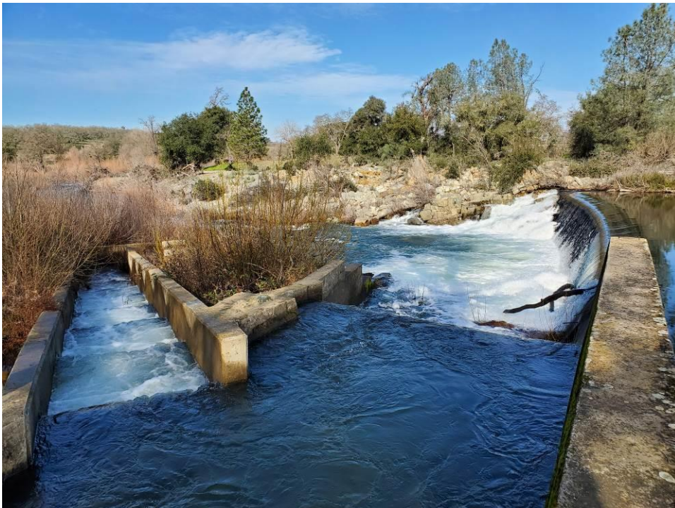
Photo 2: View of the South Dam from the left abutment looking towards the right.
