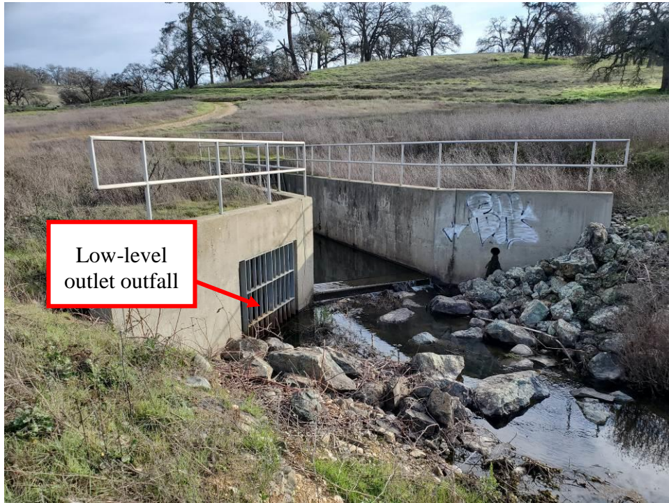
Photo 3: View of the spillway and low-level outlet outfall structure looking upstream.
