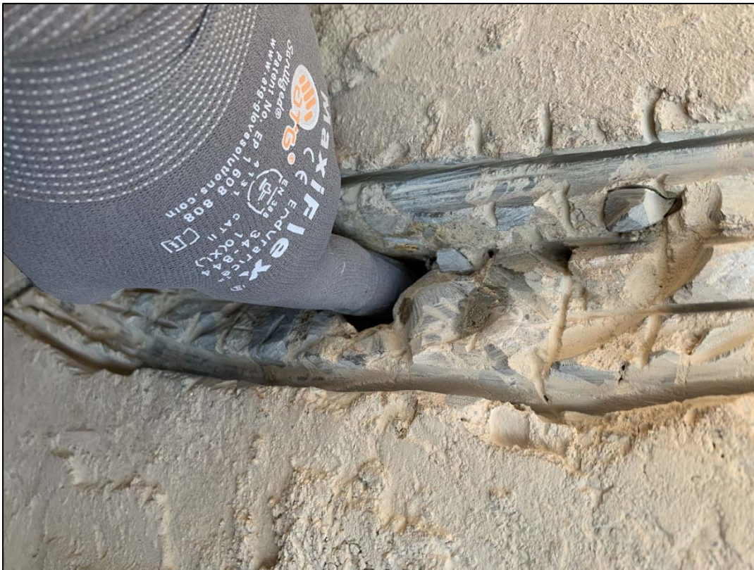
Hole in CIA diversion box next to Country Store, prepped for repair
