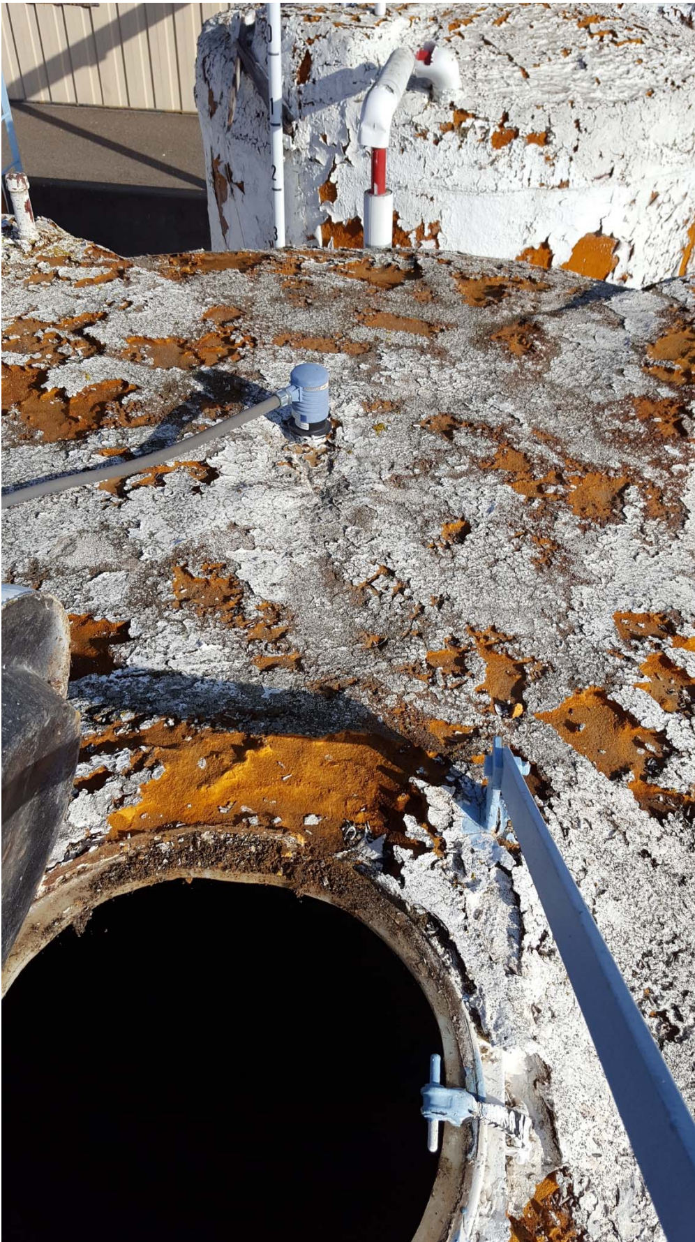
View of top of existing caustic tank with hatch open
