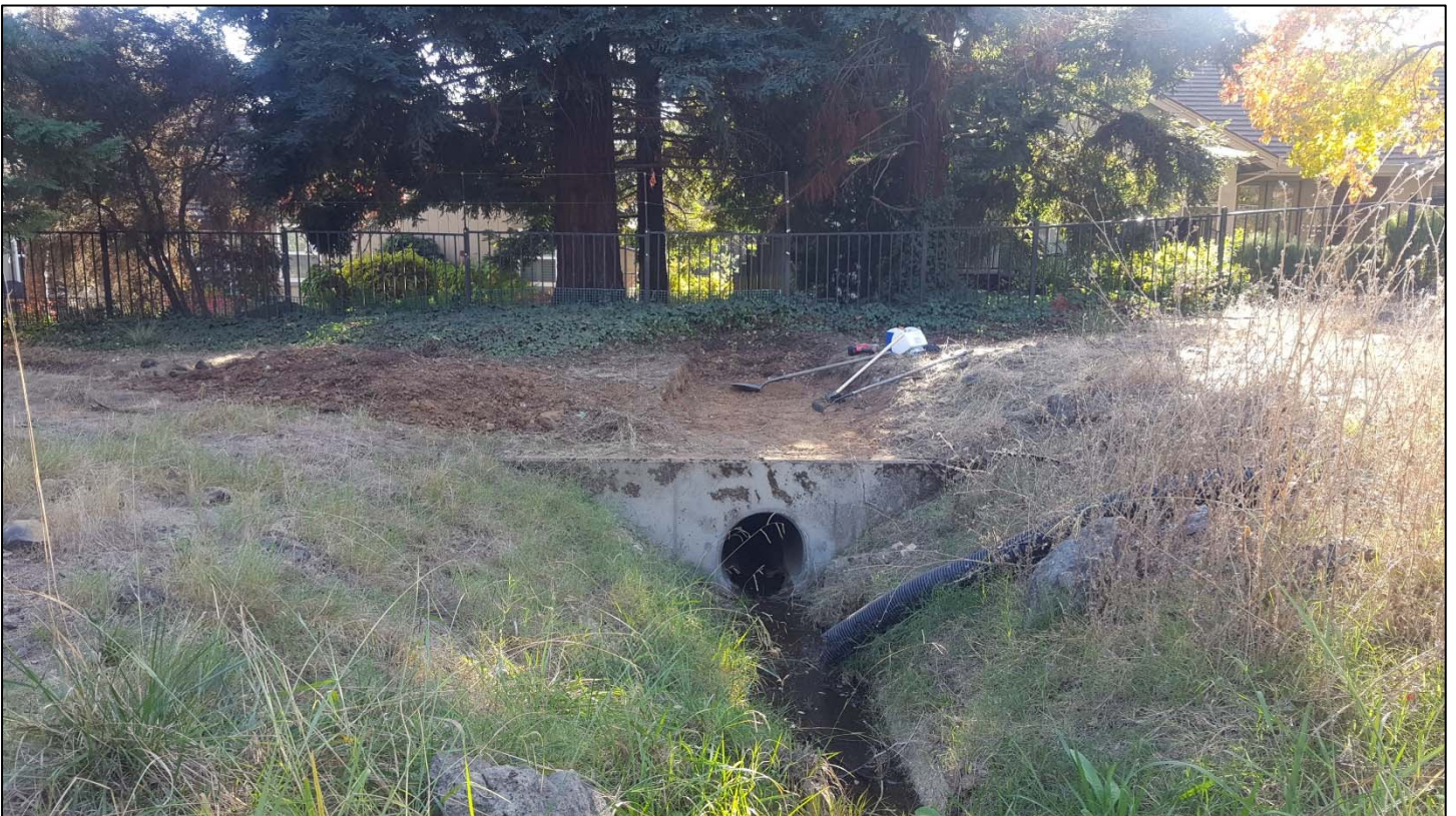
Work completed by District behind Zieour's lot as of 11/22/19.
