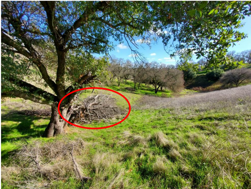
Photo 6: View of the downstream face of the North Dam from the right groin looking towards the toe. The fallen limbs shown by the red circle need to be removed.
