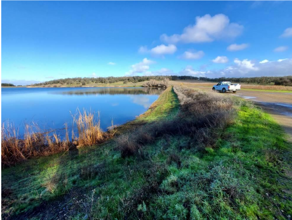
Photo 3: View of the upstream face of the East Dam from near the right abutment looking towards the left.
