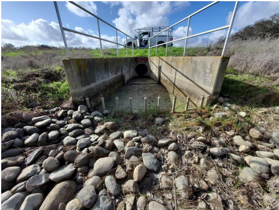
Photo 6: View of the spillway approach and control section looking downstream.
