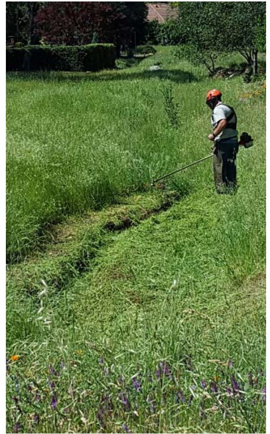
Cutting weeds in drainage
