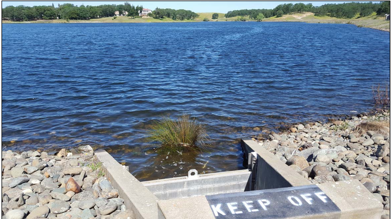
View of the Chesbro Reservoir from the spillway with "stop-log" installed
