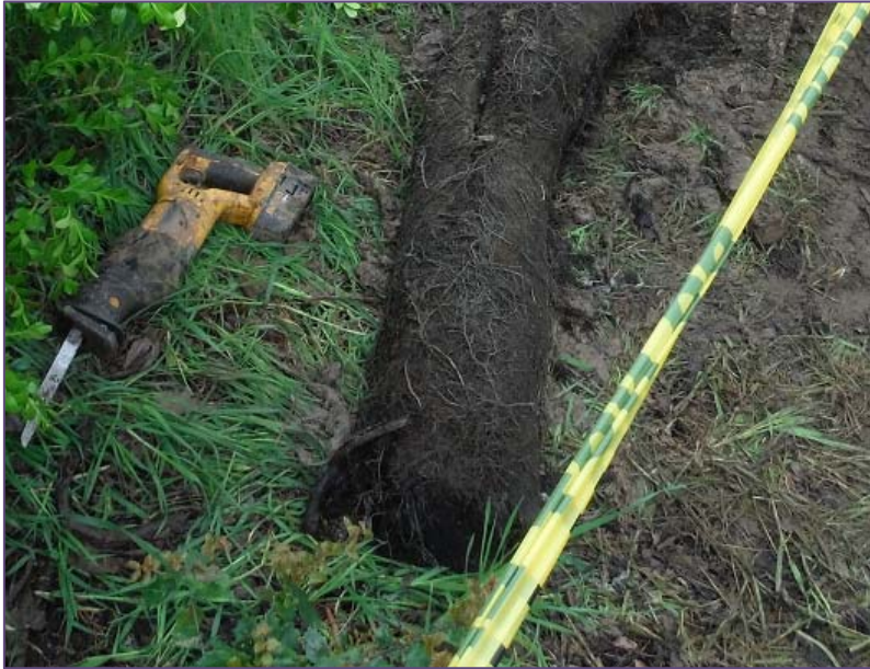
Roots removed from drainage pipe
