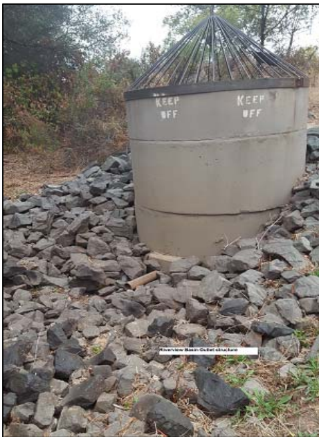
Riverview basin outfall
